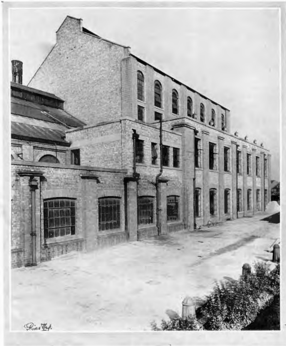
EXTENSION TO TURBINE ROOM, SWITCH HOUSE AND FITTING SHOP
