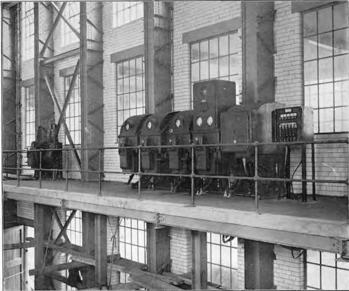
L.T. SWITCHBOARD CONTROL GALLERY
